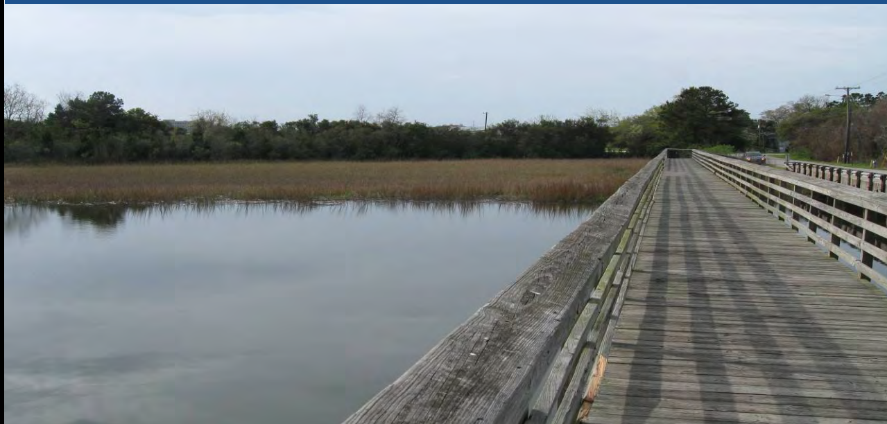
View from Bridge on O'Hear Street
