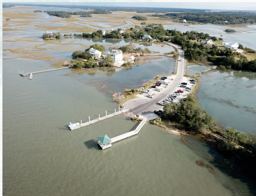
Battery Island Landing at Sol Legare - James Island
